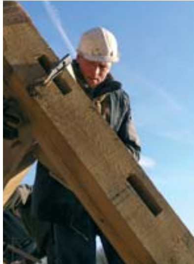
Restauration de la charpente © IPW
