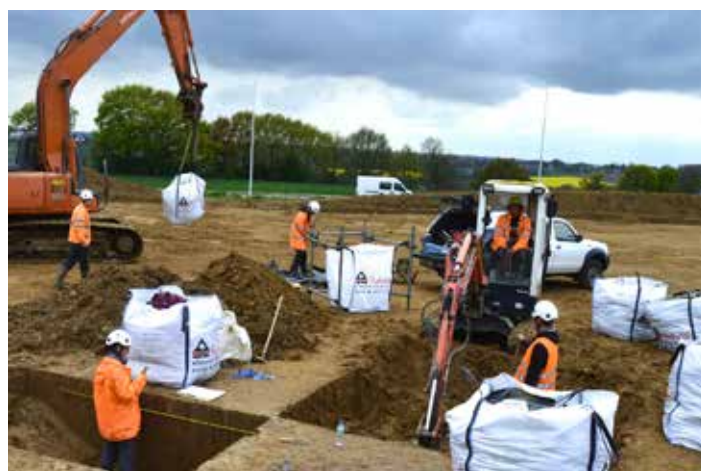
Liege Airport, Airport City 4. Tamisage des sédiments © SPW-AWap (cliché S. Denoël)
